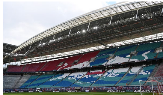
The installation of the new seating shell was carried out by a stadium seating expert during the ongoing Bundesliga match operations.
